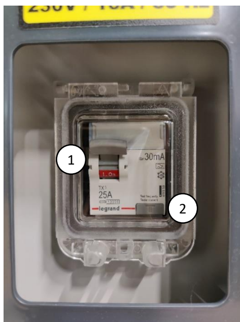
Figure 8. Residual current device
