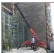
Level operation on uneven sites
